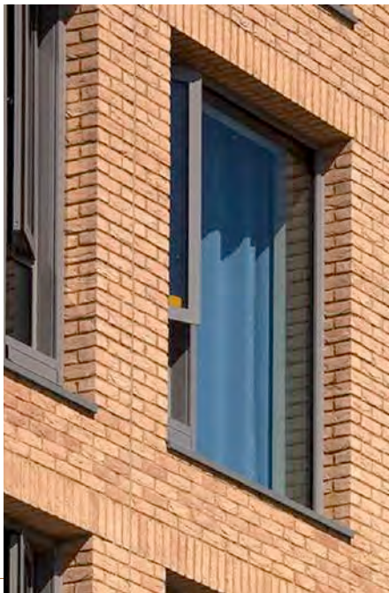
Example of windows set deep in reveal
