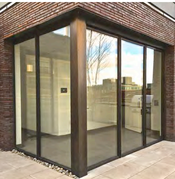
Example of dark bronze window frames to tonally complement red brickwork
